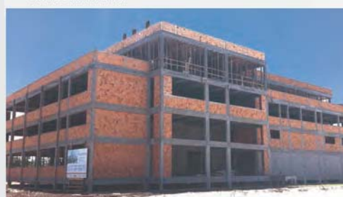
Building for the Pharmacology Center in construction phase at Sapiens Parque
